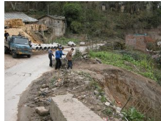
Construction phase of Magutan town
