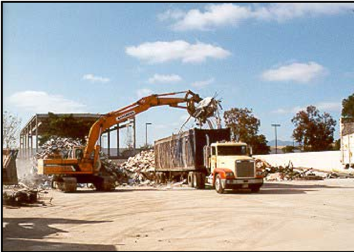
Figure II-3. Bulky metallic waste being loaded for transport to market
